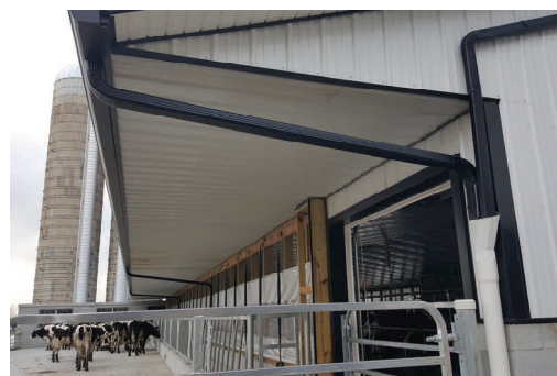
Roof Runoff Structure
