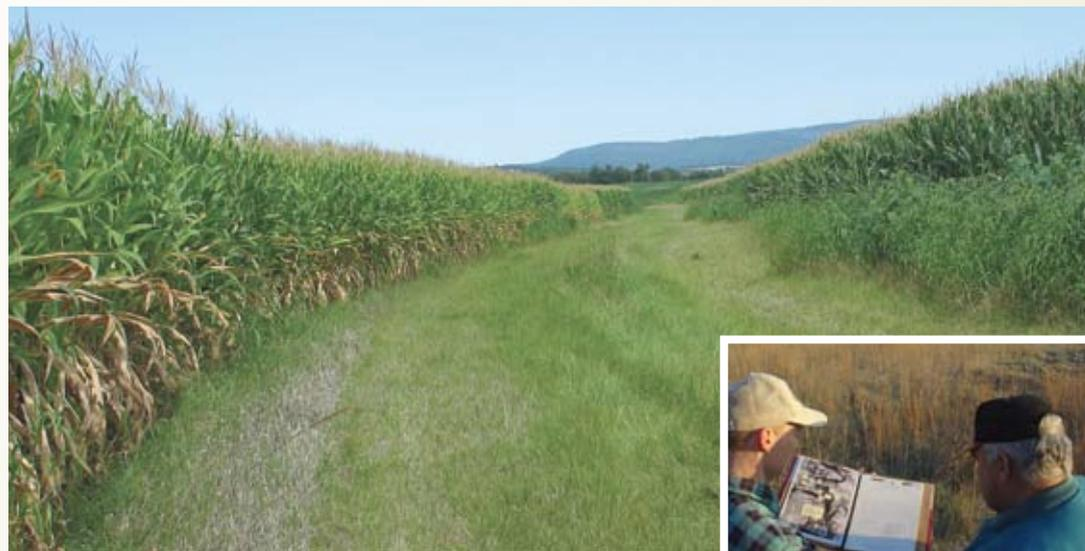
*Grassed waterways constructed in natural drainageways help prevent gullies from forming and control soil erosion.*
