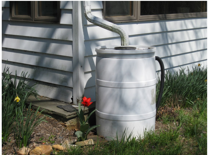
Rain barrels can be wooden or plastic. This plastic, 55 gallon drum rain barrel is located at the Fair Hill Nature Center.
